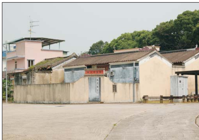
Developed Area at Tsung Yuen Ha
