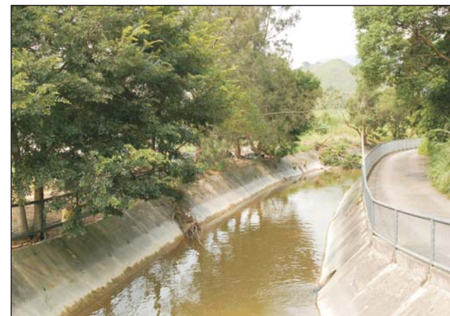
Channel at Tsung Yuen Ha
